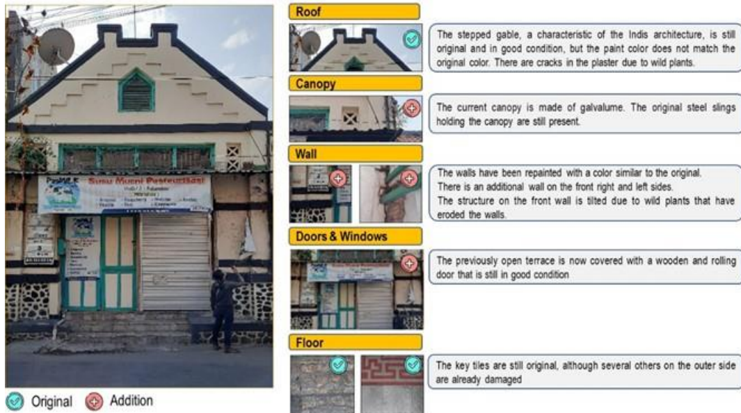
Fig 6: Identification of Facade Damage of the Kwan Nio Tio Shop House Source: Author, 2023
