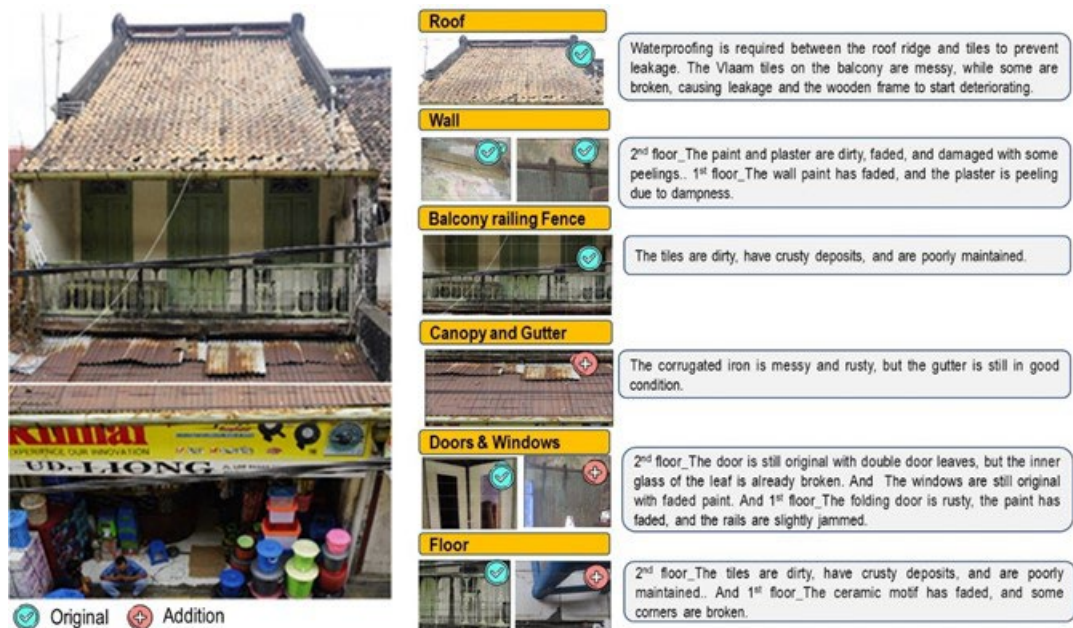
Fig 14: Identification of Facade Damage of the Liong Shop House
