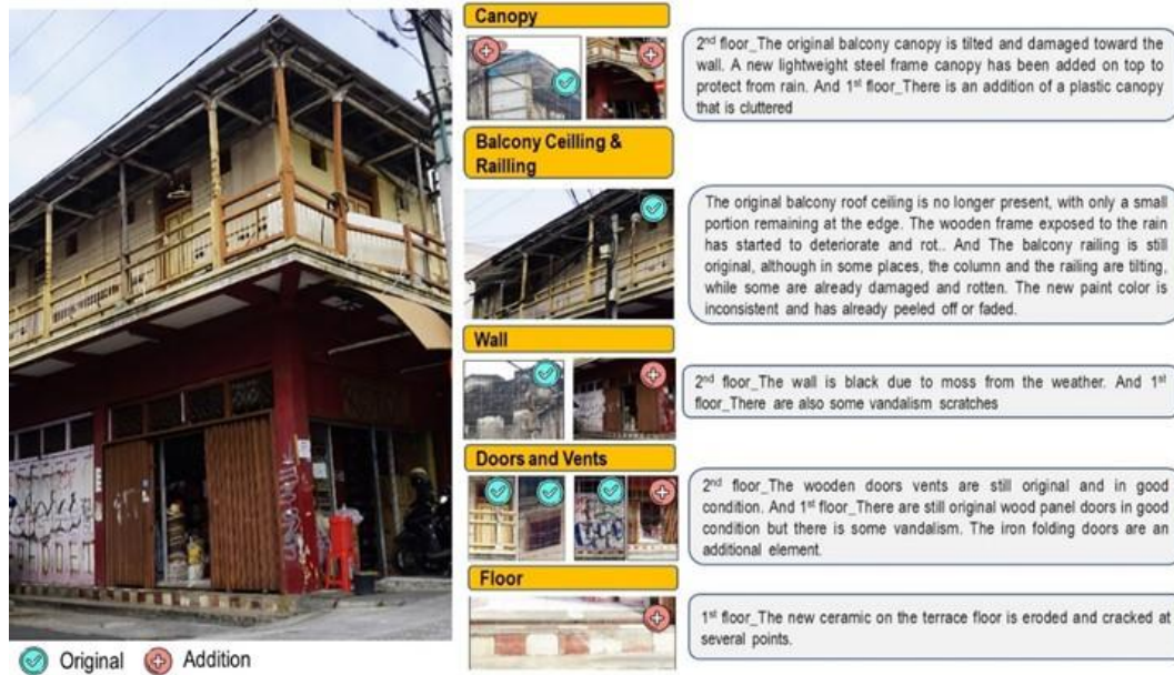
Fig 17: Identification of Facade Damage of the Windiastuti Shop House Source: Author, 2023
